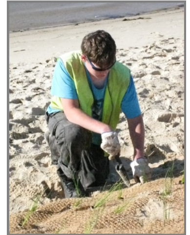
Volunteers install and plant sedges in coir matting along an erosion site at Pelican Point.
