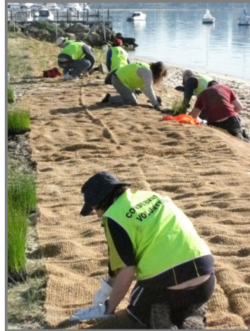
Volunteers install and plant sedges in coir matting along an erosion site at Pelican Point.
